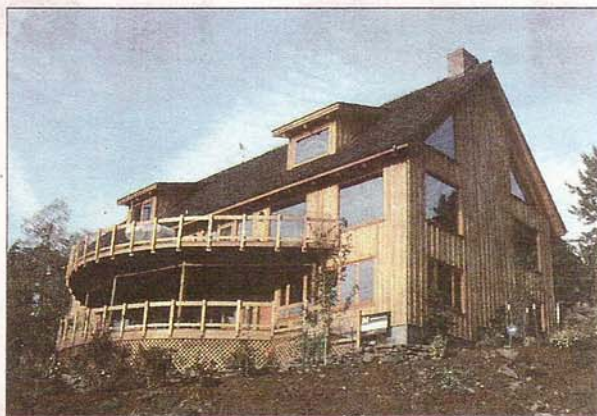
The basic shell of Roberts' 6,000-square foot home copies a timber-frame barn near Lorane. The distinctive oval decks serve the main level above and guest quarters below.
